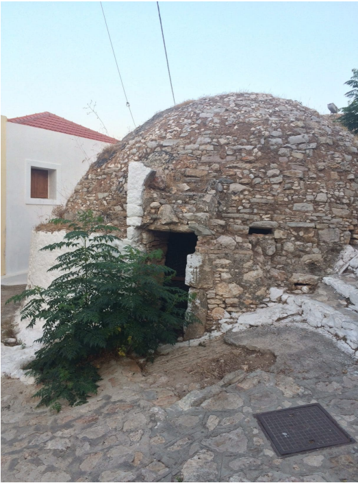
Fig.3 Kóφη (kifi), round built construction where the shepherds used to stay during spring and summer while moving with their herds. Halki, 2017 photo © Kyriaki Goni
