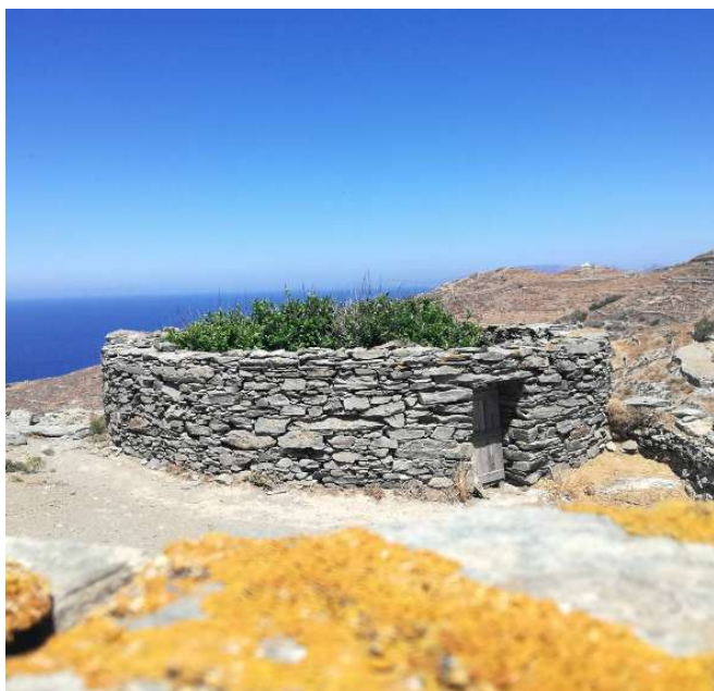
Fig.2 Περιβόλι (Perivoli or lemonhouse) built exclusively for protecting lemon trees from strong winds. Folegandros 2017, photo © Kyriaki Goni
