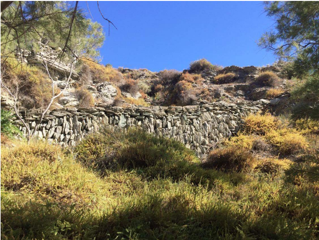
Fig. 4. Example of vertical dry wall stone. Folegandros 2017, photo © Kyriaki Goni
